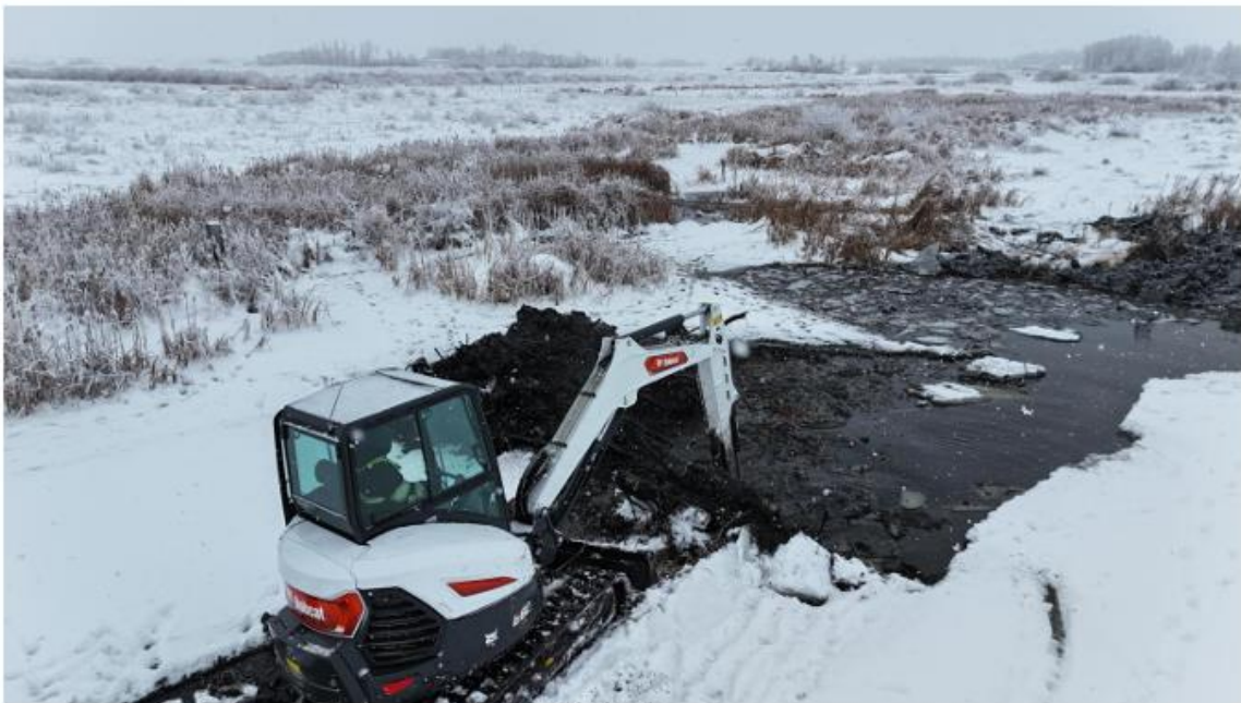
Figure 3 Removal of the secondary dam at Crescent Creek, November 2024.
